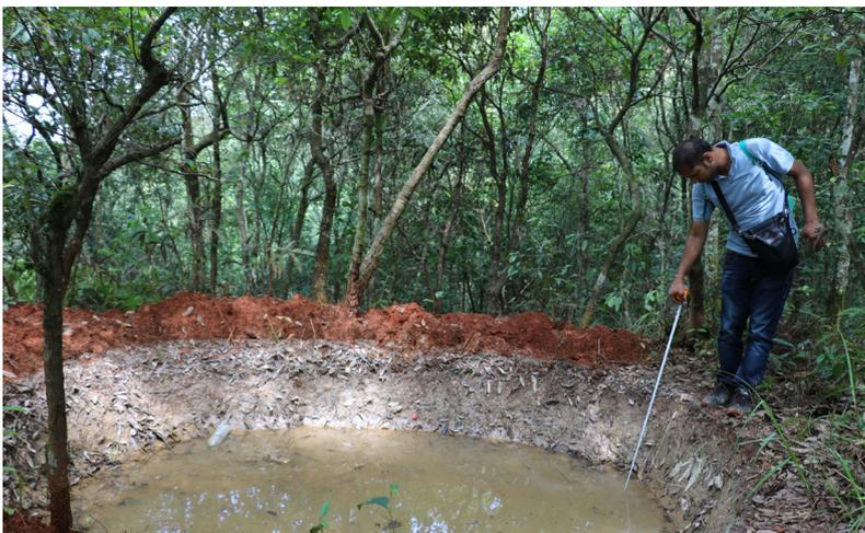
*Fig 7: Piloting recharge pond in Dhulikhel*
